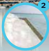
The slurry will flow in a floating pipe to a drainage area near the Pond 5 dike.
